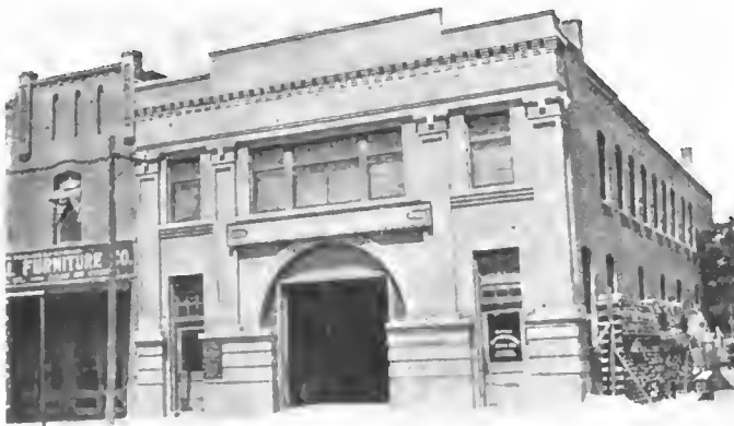
A Typical Garage Building in Ft. Worth, Texas.
